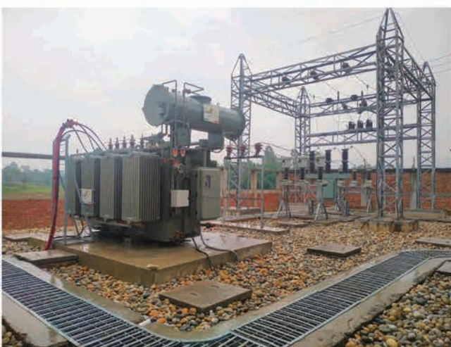
Trench cable laying at Sub-station
